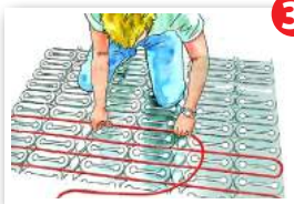
Install heating cable in grooves, pressing gently
